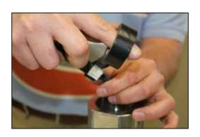
10. To ensure the connection stays together, put a few wraps of electrical tape around the connector.
